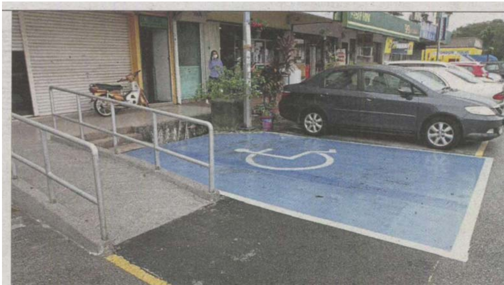
The new carpark with a ramp for the disabled in Taman Mayang Jaya.
